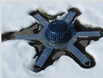
Roof/Drain De-Icing System
